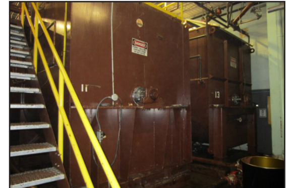
Chocolate tanks sealed with Chesterton 442C Split Seals.
