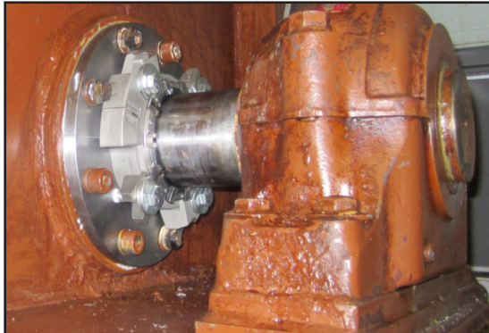
Agitator fitted with a Chesterton 442C Cartridge Split Seal.
